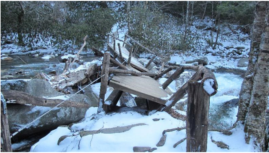
Bridge To Chimney Tops
